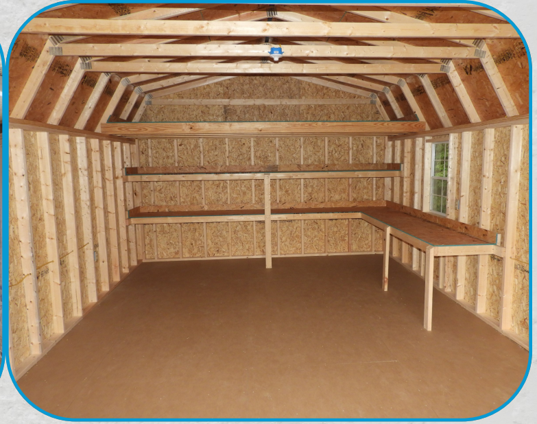
High Barn inside view w/ 4' Loft, 2' Double Shelves, 2' Work Bench
